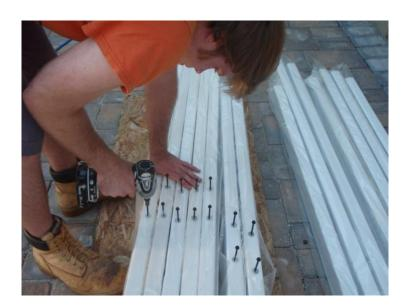
Set the screws into the predrilled holes in the rafters on the ground first. Make sure point of the screw is just in the bottom hole.
