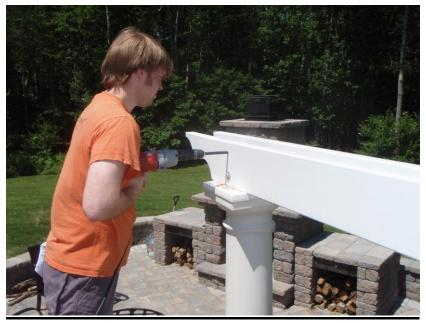
HOLD LINTELS IN PLACE AGAINST THE POST CORE WITH A CLAMP. USE EIGHT INCH LONG  $\frac{1}{2}$ " DRILL BIT TO DRILL THRU EACH LINTEL AND THE STEEL POST CORE IN A SINGLE PASS.
