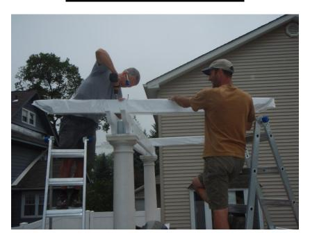
Leave protective plastic on the rafters when installing to help keep rafters clean of handprints. Set back screw first, check level and set front screw. Be careful not to overtighten.
