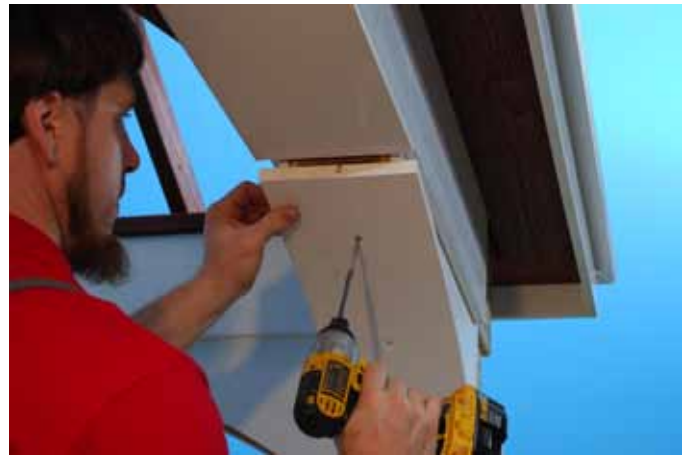
Measure reveal of Brace Cover on the inside and the outside of the Arch Brace for an equal distance.
