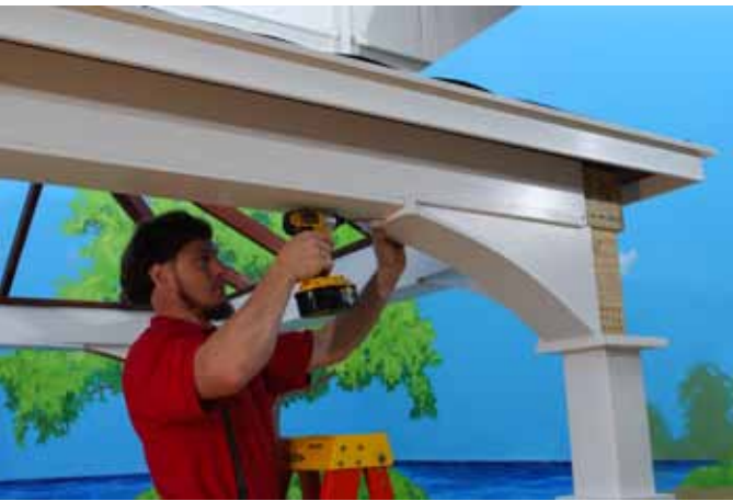
Fasten Brace Trim to Arch Brace using (1) 2.1/2" White Head Screws centered on Brace Trim.
