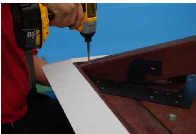
Attach with (2) 2.1/2" Brown Screws at approx 1" from end through top down.
