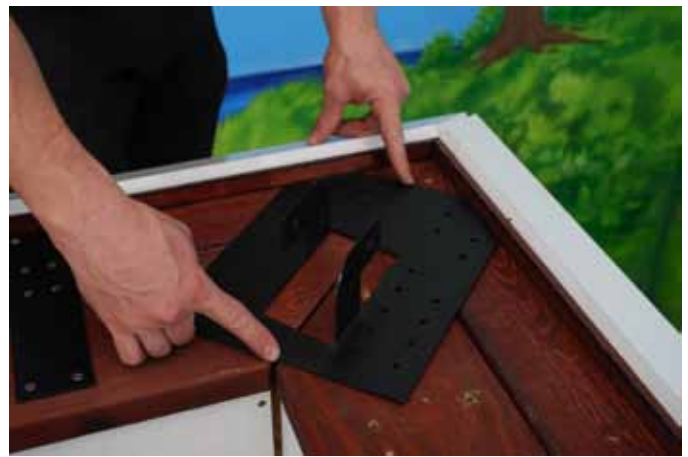
Place Corner Rafter Plate centered onto roof plate joint. Align notched section of Corner Rafter Plate with the corner of the Roof Plates.
