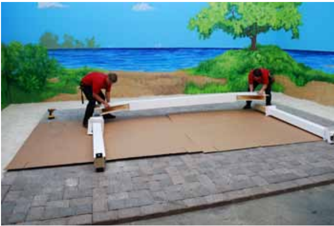
Place Header Beam & Arch Braces onto Posts.
