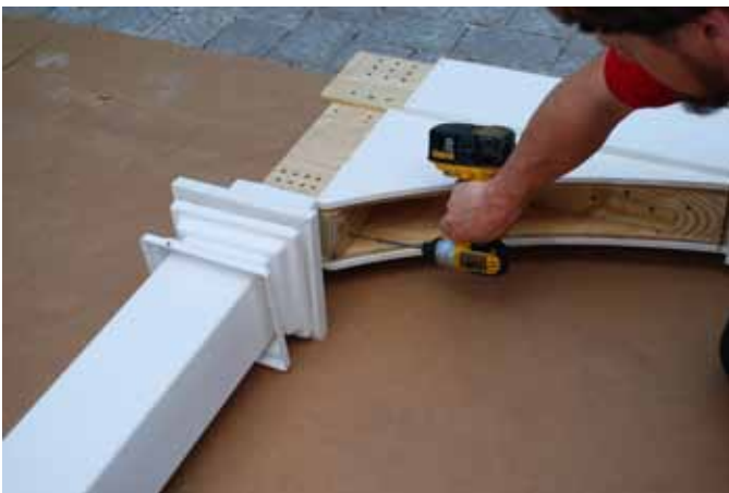
Fasten Arch Brace to side of Post using (5) 3.1/2" Brown Screws.
