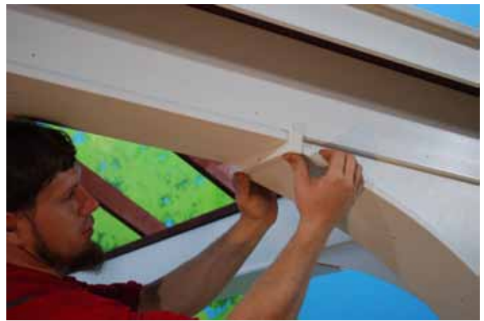
Turn groove to correct side and slide up into position.
