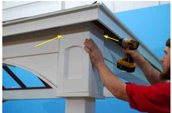
Fasten Top side of Outside Corner Cover to Headers using (2) 2.1/2" White Head Screws (1) per side.
