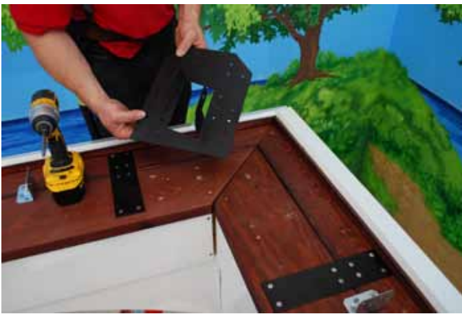
Install Corner Rafter Plate
