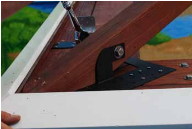
Tighten bolt on Hip Rafter with 3/4" socket.
