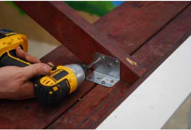
Fasten L Brackets to Single Rafter using (4) 1.1/2" screws per bracket
