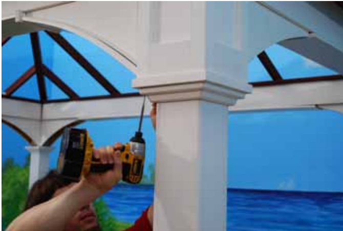
Fasten Small Trim to Square Trim from the bottom up using (4) 2" White Pan Screws
