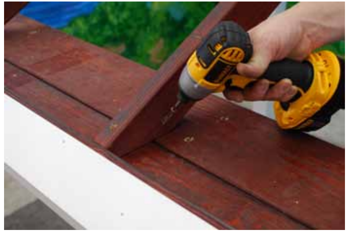
Fasten opposite side of Single Rafter to roof plate using (2) 3.1/2" Brown Screw through pre-drilled hole (Toed).
