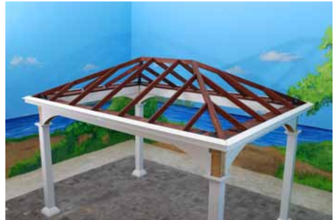
Fasten all Single Rafters as shown in prior steps..
