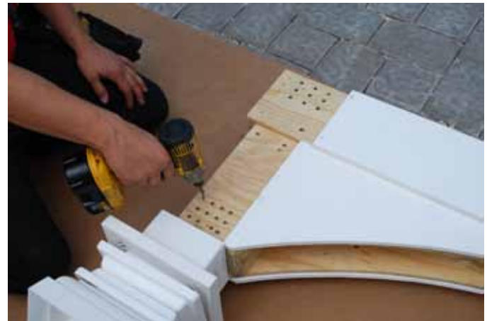
Fasten Arch Brace to Post using (14) 2.1/2" Brown Screws through pre-drilled holes. Make sure side of post is tight against side of Arch Brace.
