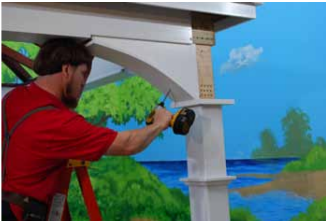
Fasten Brace Cover to Arch Brace using (3) 2.1/2" White Head Screws.
