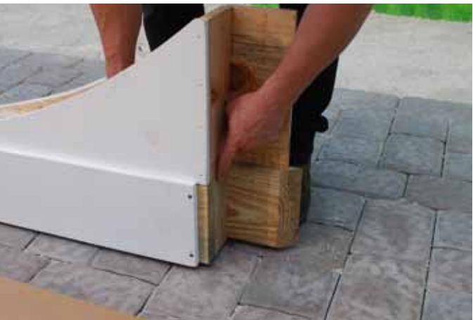
Align Arch Brace with Header Beam at the post side as shown.
