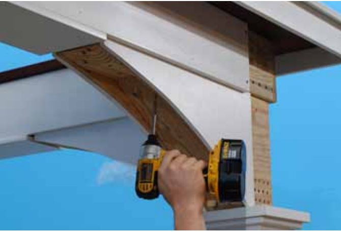
Insert brace on a 45 degree angle. Tap into place with a hammer for a snug and tight fit.
