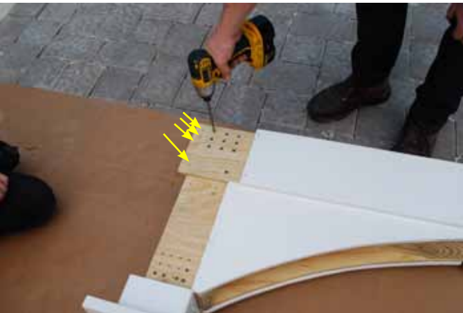
Fasten Header Beam to post using (10) 3.1/2" Brown Screws into pre-drilled holes. Do not fill the four outside holes at this time. (Shown with yellow arrows)
