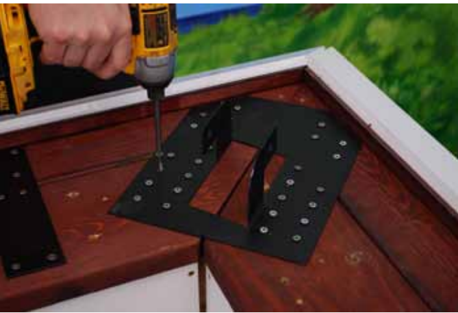
Fasten Corner Rafter Plate to Roof Plates using 1.1/2" screws into every hole.
