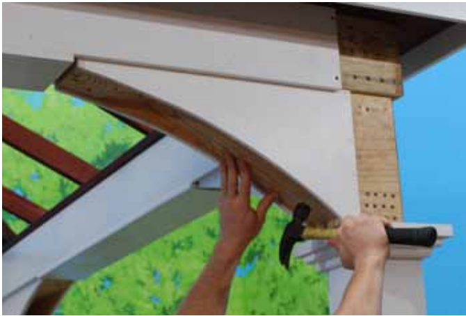
Insert brace on a 45 degree angle. Tap into place with a hammer for a snug and tight fit.
