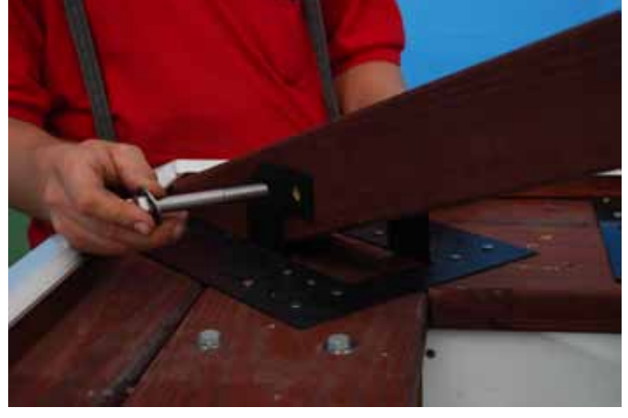
Insert 1/2" x 4" bolt and washer. Use washer and nut on threaded end.
