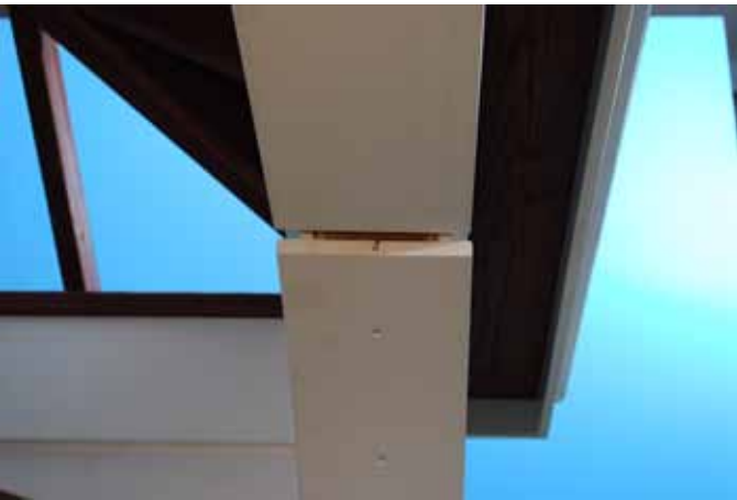
Make sure top side of Brace Cover is aligned evenly before fastening upper two screws.
