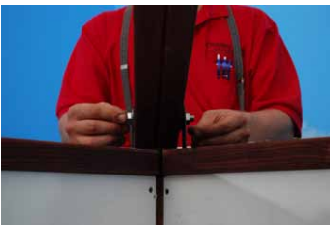
Hand Tighten Only, Leave slightly loose for easy adjustment. Note: To be tightened fully in future step. Install three remaining hip rafters.
