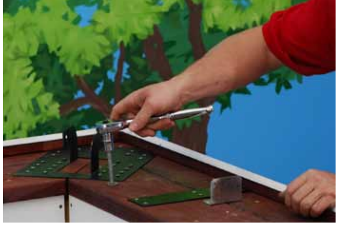
Fasten Roof Plate to Header below using a 3/8" x 3.1/2" Lag and a Washer into every pre drilled hole.
