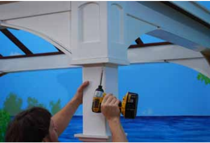
Fasten Square Trim to Outside Corner Cover from the bottom up using (3) 2.1/2" White Head Screws (1 per corner)
