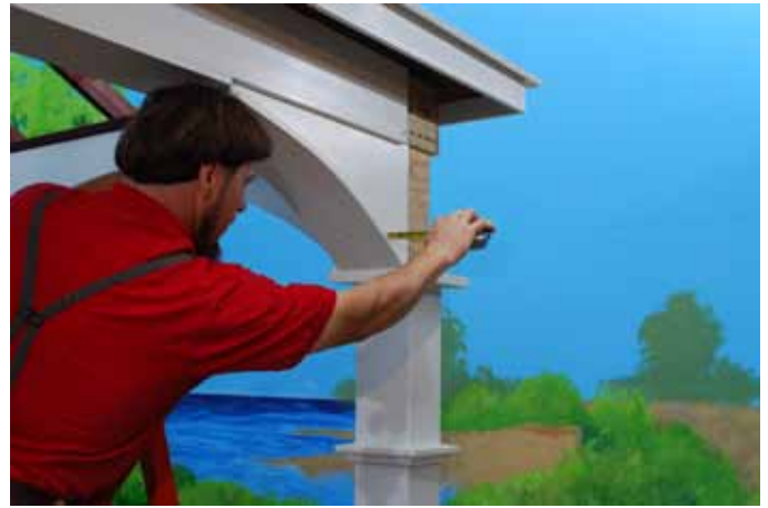
Measure reveal of Brace Cover on the inside and the outside of the Arch Brace for an equal distance.
