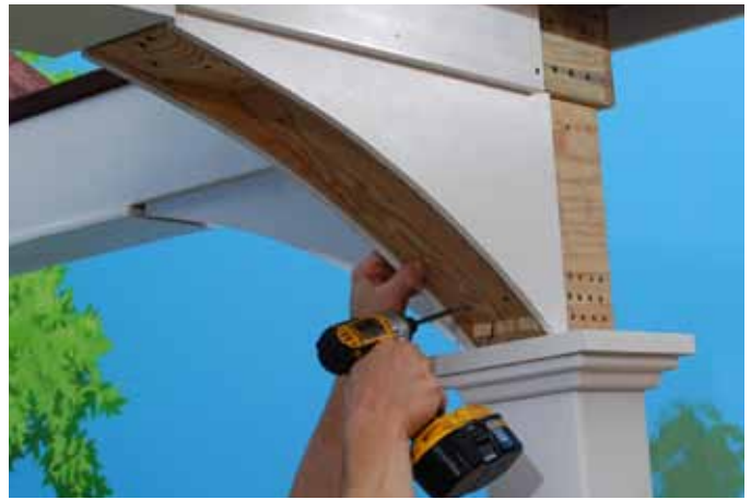
Attach using 3.1/2 Brown Screws in each pre-drilled hole. Using longer 4" drill bit will make this step easier.
